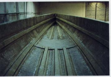
These are the continuous longitudinal stringers that provide support for the hull shell. The continuity of the stringers eliminates "hard spots" which create high concentrations of stress. The raised area across the centerline is a 3" thick solid fiberglass layup that carries the loads imposed by the keel.
